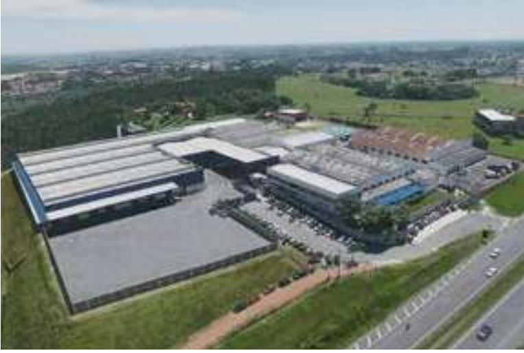
PLANT LOCATED IN ITU - SP
